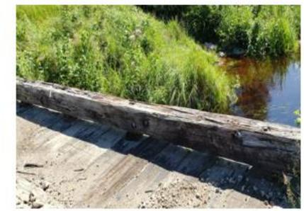
Photo 4: Splits, checks and rot on NW timber curb
