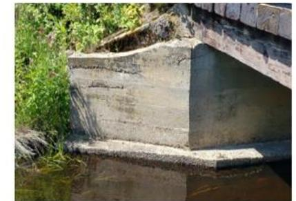
Photo 6: Moderate scaling noted on NW wingwall
