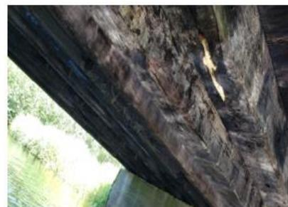
Photo 5: Weathering on timber girders
