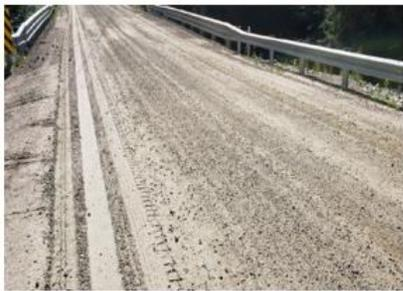
Photo 5: Tire rutting noted on east approach wearing surface
